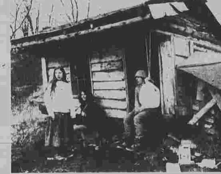
Students at the Vershire (Vt.) School, a small private prep school, were ordered by the Vermont Commissioner of Labor and Industry to vacate their rustic cabins following a fire in one of the dwellings which injured two students Saturday morning. The students are members of a wilderness program at the school which rewards high grades by the pupils by allowing them the option of living in the wood-heated cabins.
